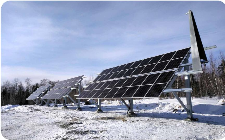
A 2021 research project, a collaboration between Bell, Québec-based solar energy company Stace and Université de Sherbrooke, studied the viability of these solar voltaic cells to generate renewable energy to provide primary power for remote telecommunications towers – displacing diesel generators and reducing the associated greenhouse gas emissions.
